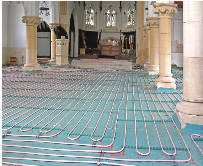
Underfloor heating being installed at St Mary's Church Loughton.
