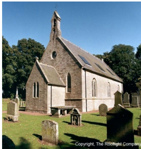
Conservation roof lights at Wiston Church, Lanarkshire (residential conversion) Copyright: The Rooflight Company
