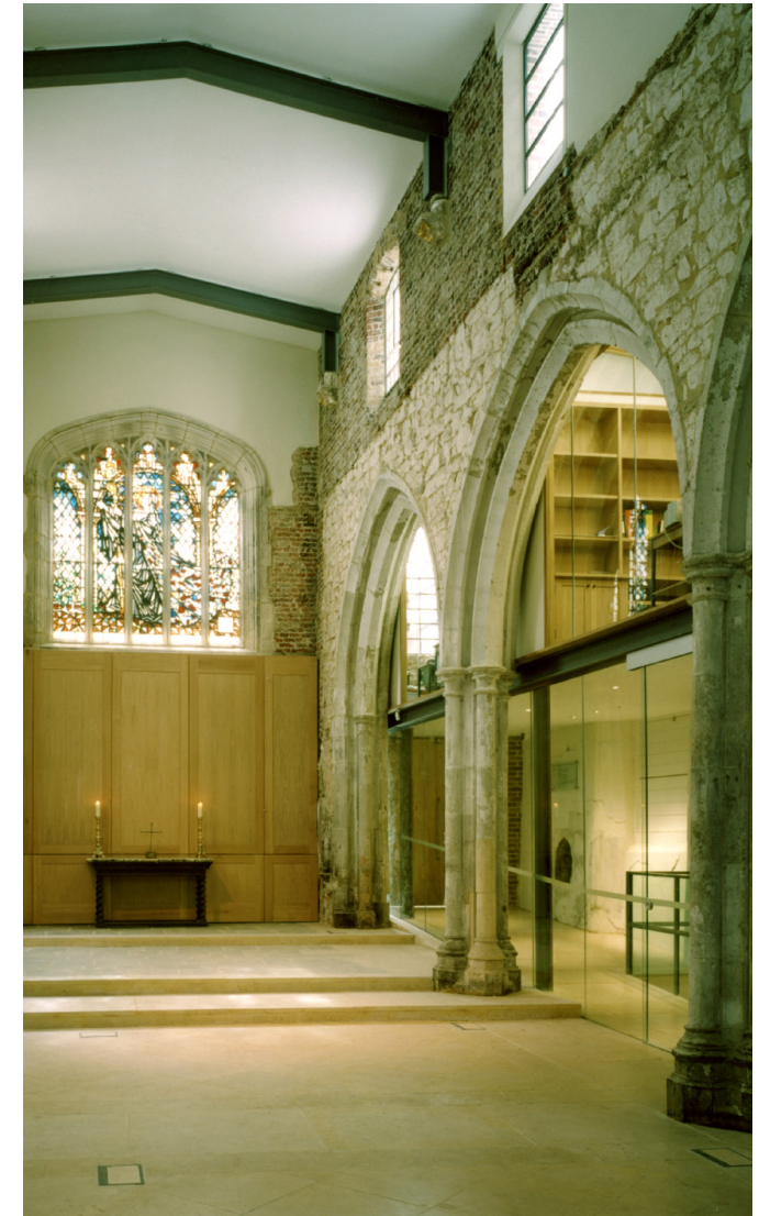
Glazed screen behind arched colonnade at St Ethelburga's Centre for Reconciliation & Peace
