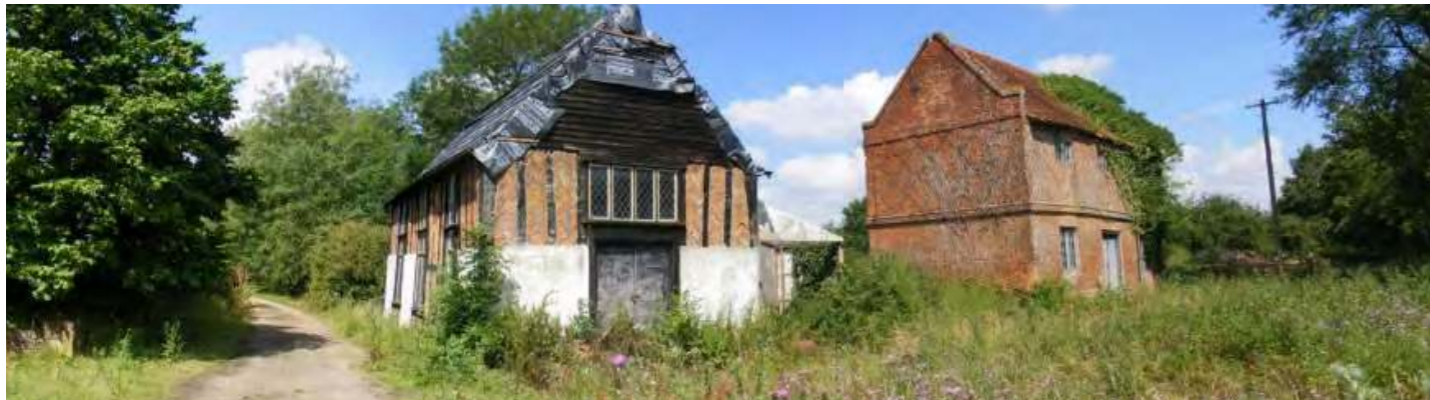
4 The chapel and barn at Marks Tey Hall.
