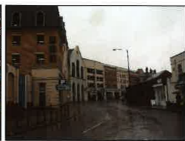
Photo 31 NCP multi-storey car park, Osbourne Street.
