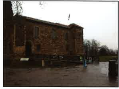
Photo 7 Castle Museum entrance bridge.
