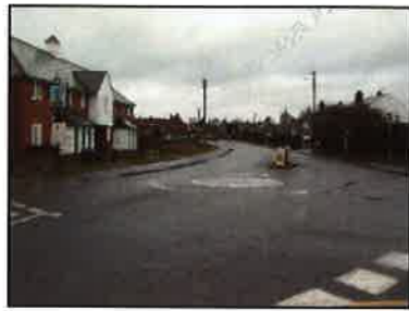
Photo 175 Looking north up Colchester Road from Wivenhoe Cross.
