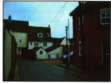
Photo 127 Nunn's Road Alley to North Hill.
