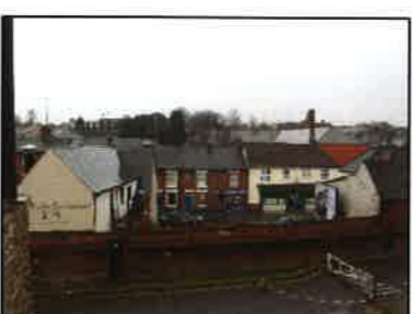
Photo 71 Vineyard Street - looking south west from Vineyard Steps.
