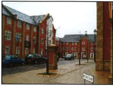
Photo 101 New Housing at Hesper Road off Hythe Quay.
