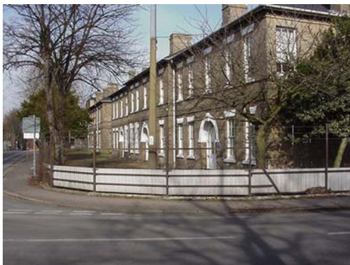
Buildings facing Flagstaff Road
