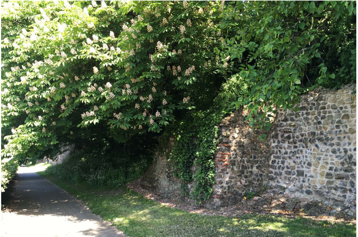
Photograph 14: Town Wall along the northern part of Balkerne Hill showing mature horse chestnut trees on the inside of, and overhanging, the Wall. Damage can be caused both from the roots of these trees and also from branches within striking distance of the Wall (May 2018)
