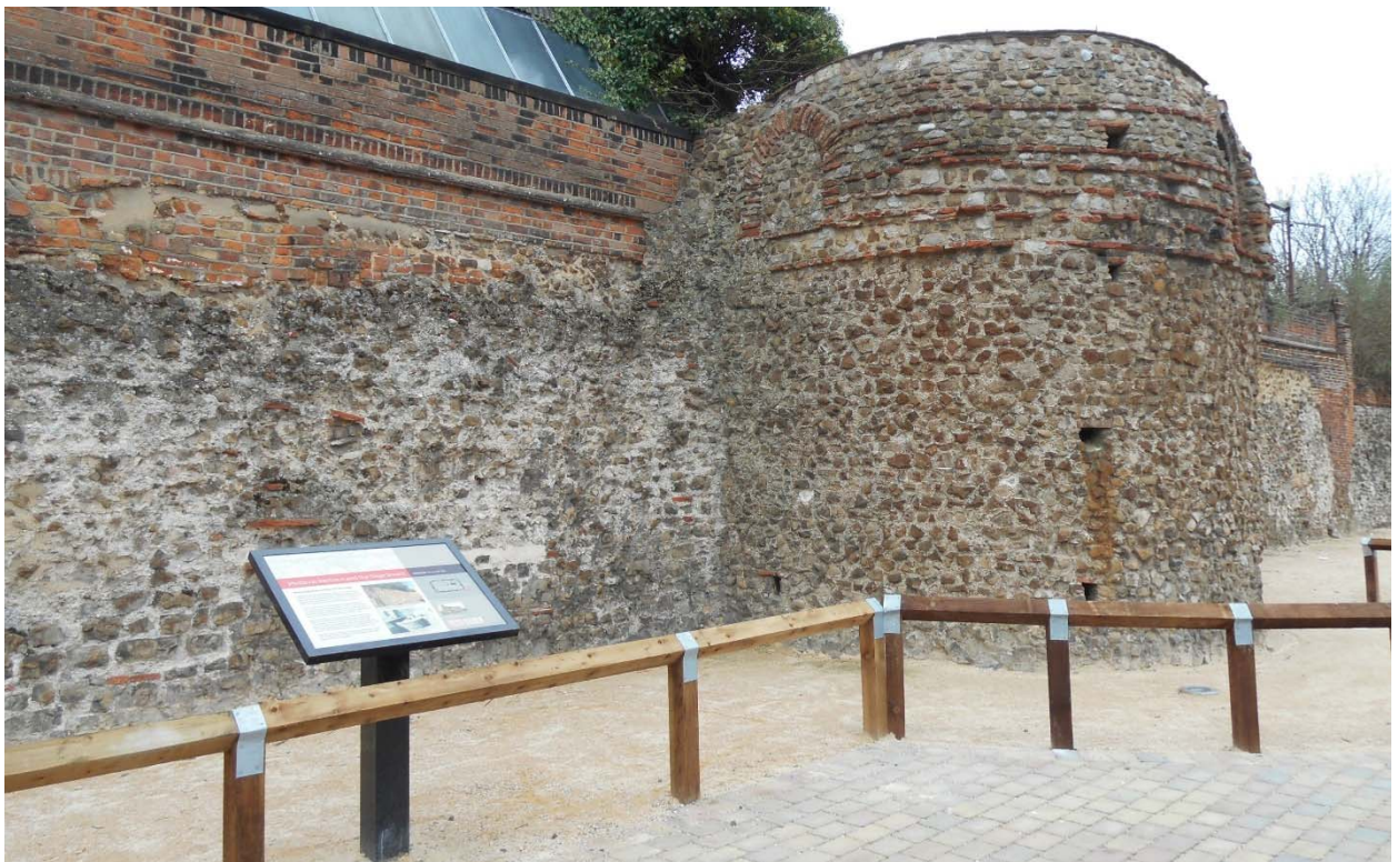
Photograph 8: Priory Street car park and Bastion 5, following car park improvements in 2017. Car parking has been removed from the base of the Wall to better reveal the significance of the Wall and also to prevent damage from vehicles (March 2017)
