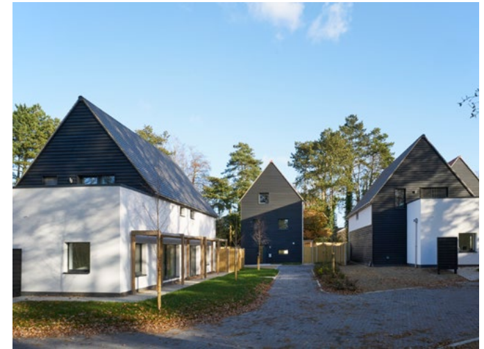
The form of these new homes draws from local rural typologies, with a contemporary interpretation. Carrowbreck Meadow, Norfolk
