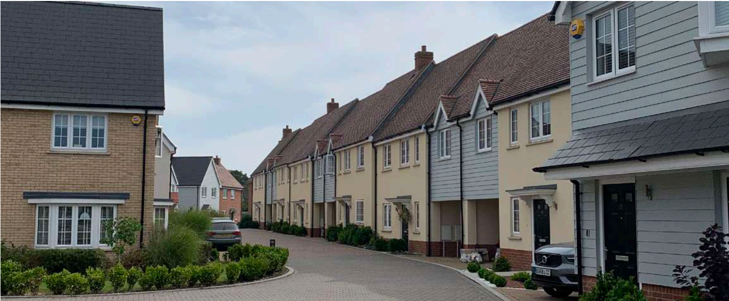
Details within this development include Splayed brick headers, stone cills, brick plinths, angled first floor oriel windows and bay windows (limited). The brick used varies between red and buff, though the use of buff brick is limited. The render colour used is also limited to yellow and cream, weatherboard is used more prominently in this development in a blue/green tone.
