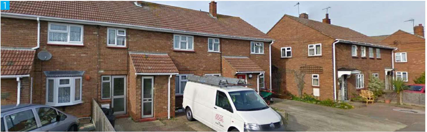
Brick Houses. A common house typology in the Northern end of Tiptree. These brick houses are commonly featured on linear streets in terraced and semi-detached forms. Front to back roofs, soldier course and tile creasing detail to windows. No other notable detailing.
