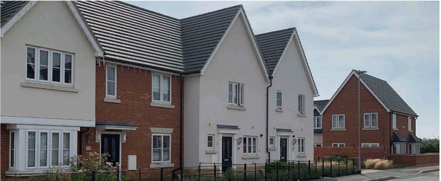
Details include splayed stone headers and stone cills, arched brick headers, dummy windows, brick plinths, projecting gables, bay windows. Additionally the brick used varies between red and buff, render colours also vary between pastel tones however there is, as can be seen above random application of bright blue render which negatively attracts focus from the rest of the street scene. Weatherboard is deployed however it is used sparingly.
