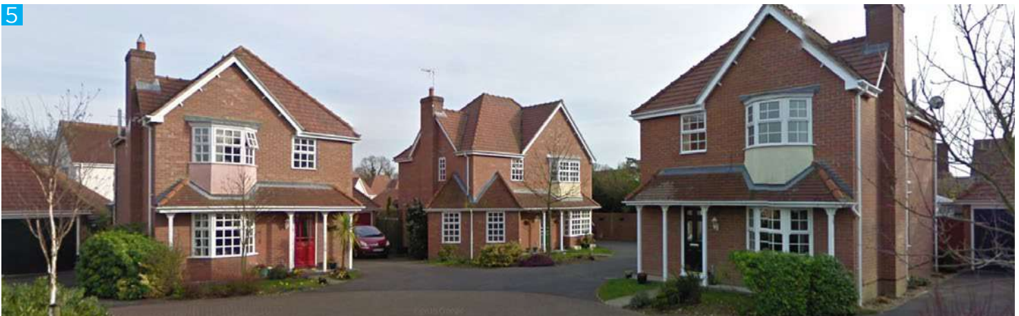
Mill Close. A recent development of 5 new dwellings all served by a private drive. Brick built, with interesting ground floor corner features, double height bay windows with varying render colour finish. Columns supporting porches provides a level of grandiosity as do multi bar casement windows and chimneys.
