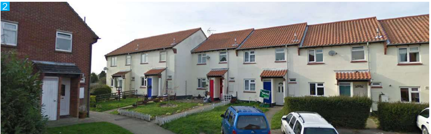
Render Houses. Similar to the Brick house typology also found in the Northern end of Tiptree though only feature in this cul-de-sac on Chestnut Way. Front to back roofs, tile creasing detail to windows, and brick corbelling utilised. Storage area to front of dwellings. No other notable detailing.
