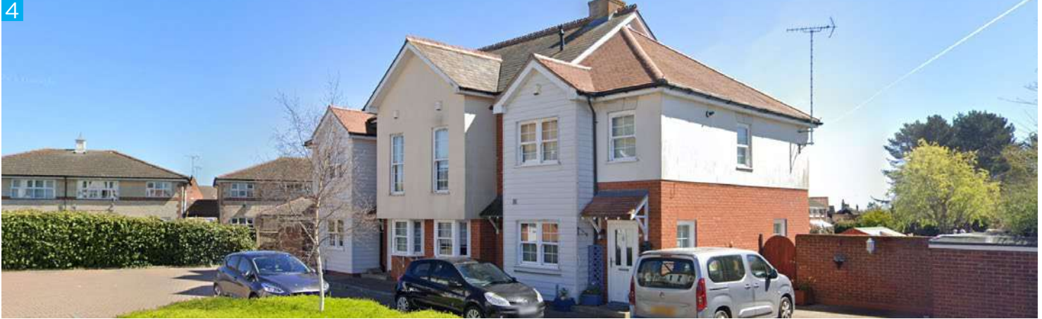
11-14 Kelvedon Road. A relatively new development of dwellings south of the Application site. Featuring an enthusiastic use of multiple materials, including weatherboarding, different render colours, brick, 2 different roof tile colours and types and brick and stone detailing to window heads and cills. Resulting in a busy, cluttered elevation.
