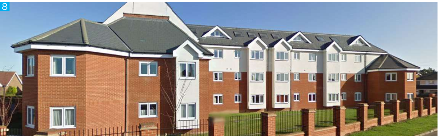
Over 50's Development. Large scale development of 1 and 2 bed apartments for over 50's spread across 3.5 storeys. 2 and 3 storey projecting gabled bays add visual interest and break the roof line. Octagonal corner elements also feature. Materiality is simple, brick and render used, arched brick headers applied to windows.
