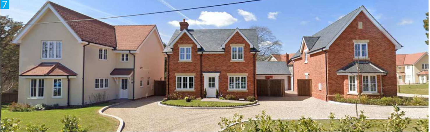
Maldon Road. New development of 7 large dwellings located on Maldon Road. Cleanly finished, features a mix of fully render or brick houses, with additional features such as wide bay windows, stone window head and cill details, stone gable features and brick plinths. Gablets used to create varied eaves line and add visual interest.
