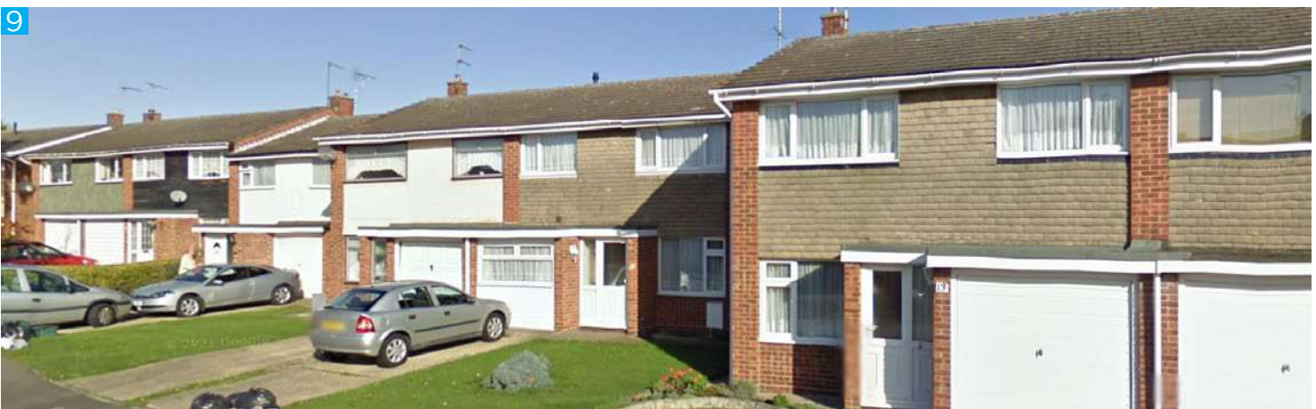
Millwrights. A very common building typology featured in many towns and villages. Brick piers provide visual separation between otherwise terraced/semi-detached dwellings. Ground floor typically finished in brick with first floor either render, tile hanging or weatherboard. Windows are typically large and uPVC.
