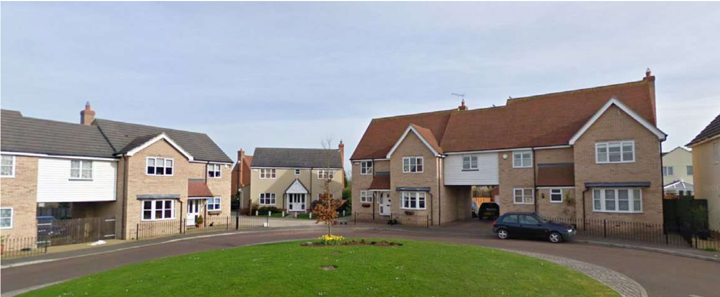
Details within this development include soldier course headers, stone cills, brick plinths, string courses, projecting gables, bay windows and gable brick features. Additionally the brick used varies between red and buff with some instances of different red bricks being used to accentuate details such as headers or string courses. As has been discussed render colours also vary between numerous pastel tones which creates a colourful and vibrant streetscene. Weatherboard is deployed however it is used sparingly for flying links or porches.
