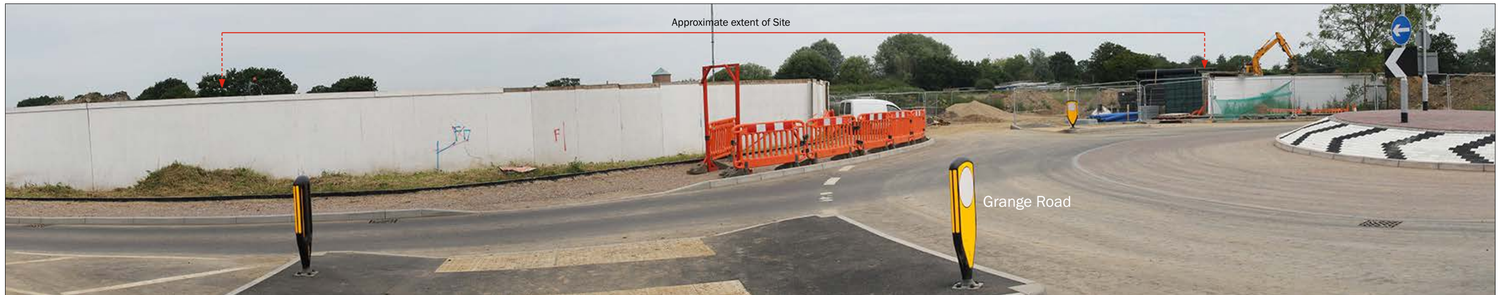
Photo Location 8: View looking north west towards the Site from Grange Road.
