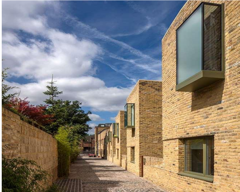
Moray Mews, London – Part-frontage to alley with obscured glazing protecting neighbour privacy
