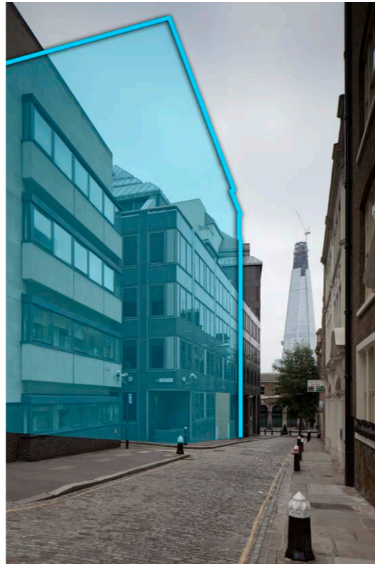
AVR0 Showing location and size (in this case as a toned area superimposed on photograph)
