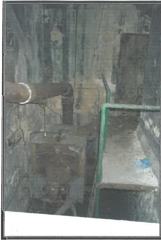
VIEW FROM WINDOW INTO BOILER ROOM
