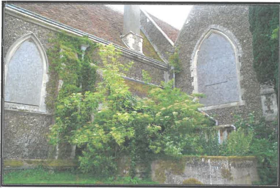
EXTERNAL VIEW OF BOILER ROOM AND TANK WHERE OVERGROWN
