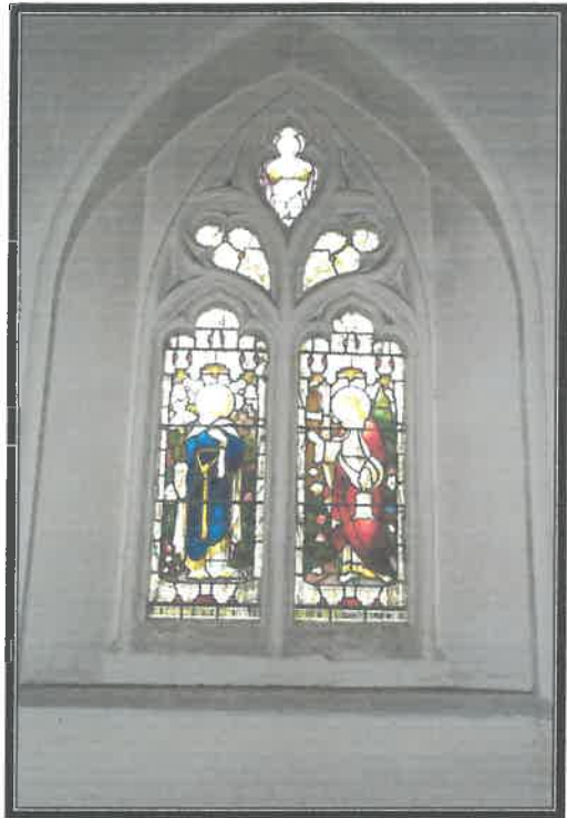
UNPROTECTED STAINED GLASS WINDOW
