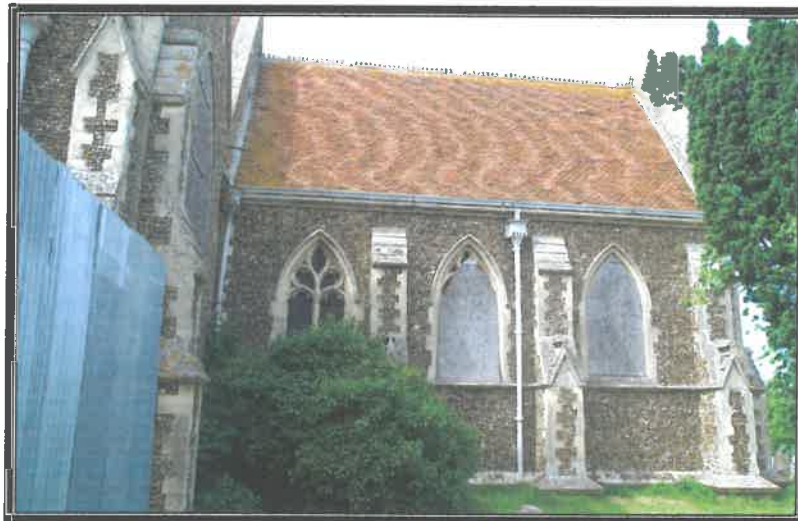
EXTERNAL VIEW OF CHANCEL FROM RIGHT HAND SIDE
