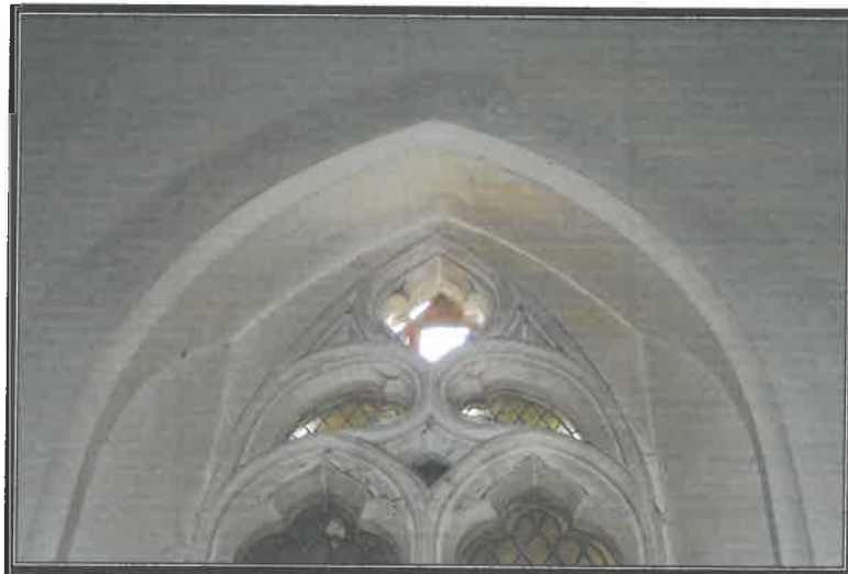
EXAMPLE OF DISCOLOURED WALL INTERNALLY
