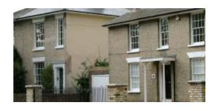
Often their use was confined to the facade with the side and rear walls being constructed in cheaper red stocks. Buildings constructed with these bricks are a familiar part of the North Essex rural and urban scene.
