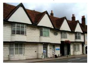
In the 18<sup>th</sup> century it became fashionable to remodel the front of medieval buildings in a classical style by constructing a façade with a parapet gutter and stucco finish. There are several examples to be seen in Dedham
