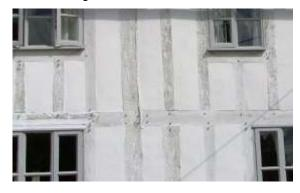
This was used as a protective coat on buildings of timber framed construction. It was usually either limed white or colour washed.
