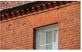
Soft red "rubbers" and lime putty were used for arches. Over burnt bricks were sometimes employed to create patterns in the brickwork.
