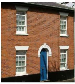
These were laid in a variety of bonds giving a rich textured appearance. Until the latter part of the 19<sup>th</sup> century they were normally pointed in lime mortar.
