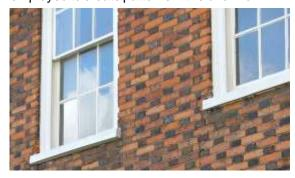
Blue and dark red engineering bricks imported from the Midlands were used in situations where strength or robustness was required such as for arches, at corners and for retaining walls.
