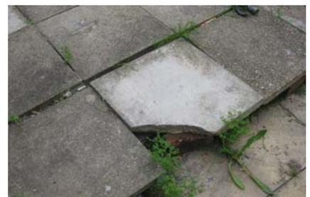
Surface variations of 5mm to floors and 20mm to paths and yards increase the likelihood of a trip. The possibility of a slip occurring is affected by both the slip resistance of the floor surface and the characteristics of any footwear. Slip resistance is worsened when a surface is damp or wet, which may be the result of a building deficiency, or be due to the purpose of the area in question, for example: kitchens, bathrooms and utility rooms.
