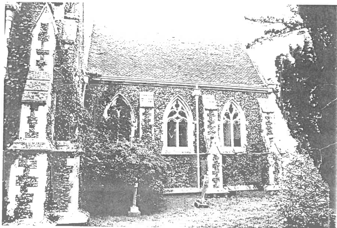
South side of Chancel.
