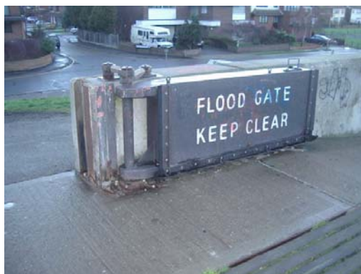
Plate 5-6 Open floodgates in Essex allowing access to and from the sea wall
