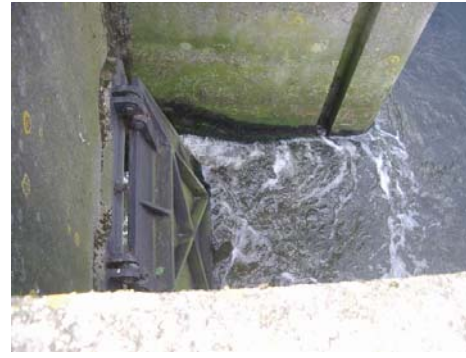
Plate 5-8 Culvert through a flood defence wall. Outlet is fitted with a non-return flap to prevent backwater effects during high tide events
