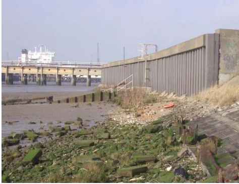
Plate 5-4 Example of sheet pile wall as a primary flood defence
