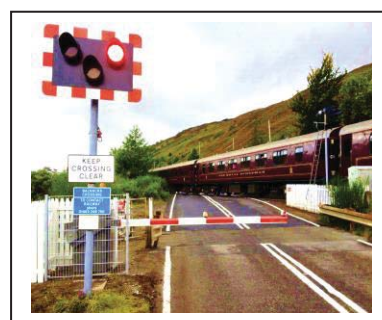
Barrier overlay installed at a significant proportion of automatic open crossings across
