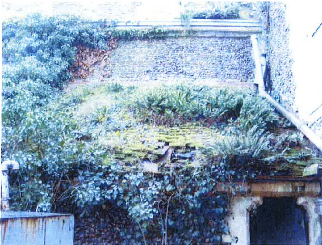
Image 02: The boiler house roof
