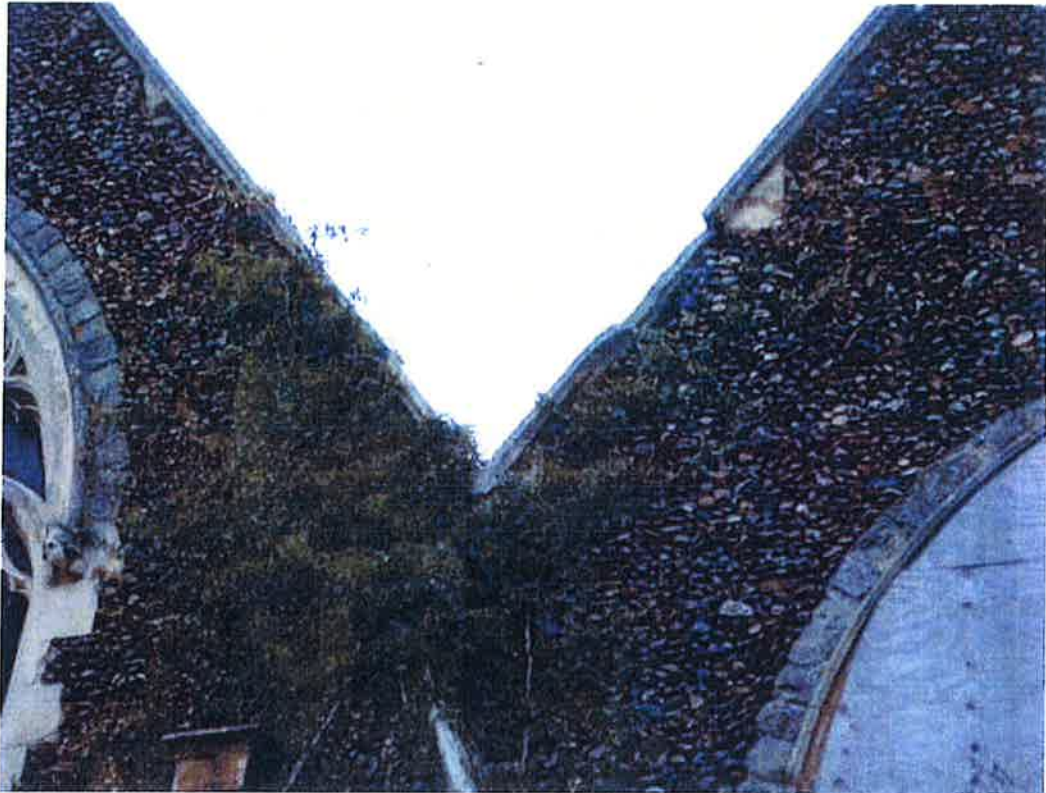
Images 09 and 10: Damage to flint and stone work
