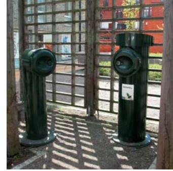
Image 79 Domestic waste chutes to underground storage, Malmö
